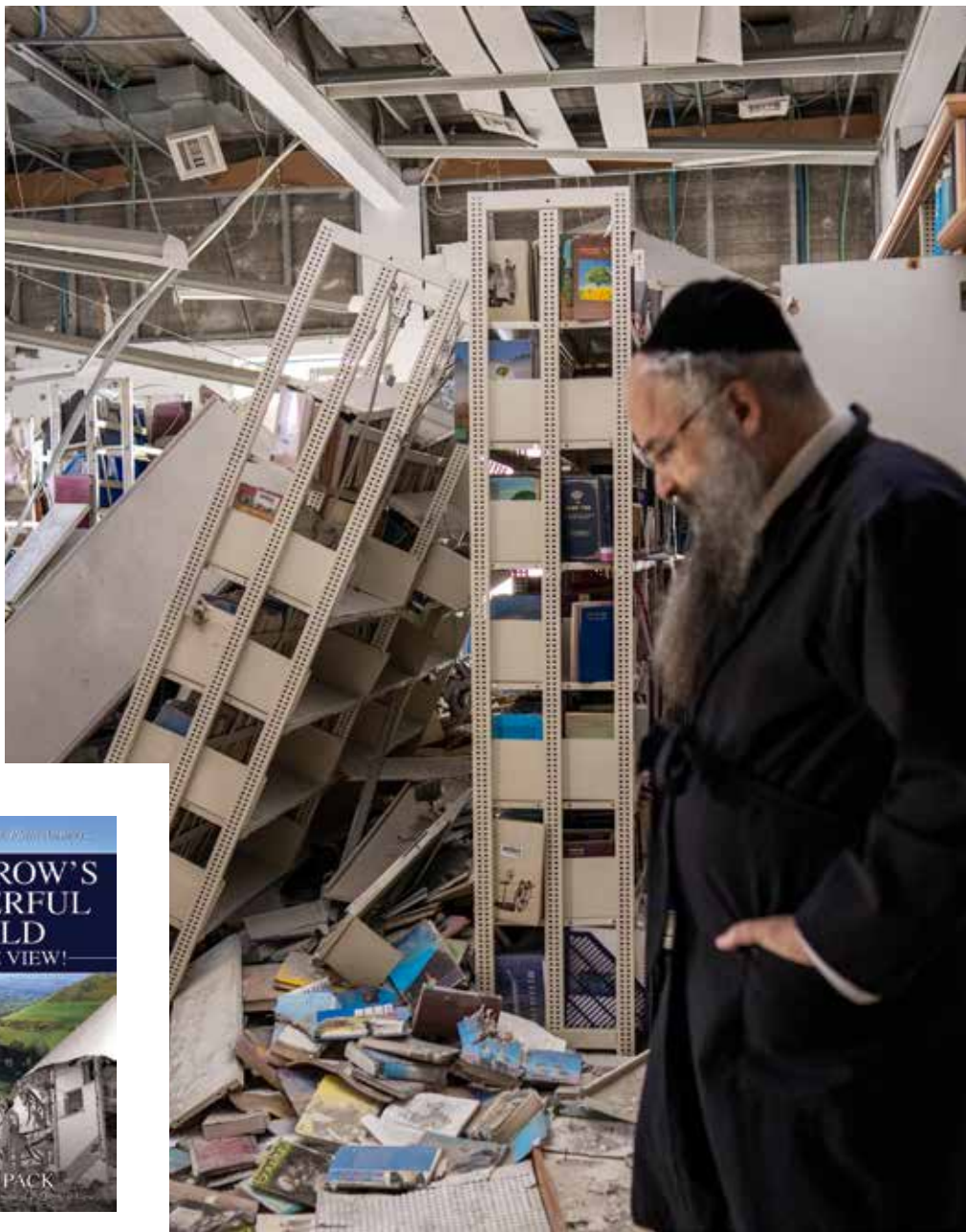
People survey the damage following an Iranian missile strike on the Beit Ya’akov girls’ high school in Tel Aviv, Israel (April 6, 2026).
